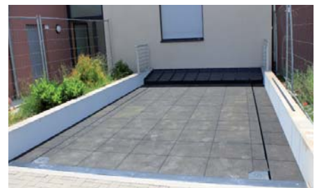
Rubber covering in stone structure (3 cm thick)
