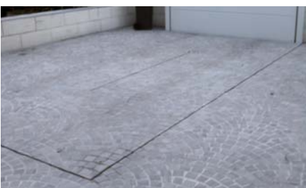
Synthetic stone covering (3 cm thick)
