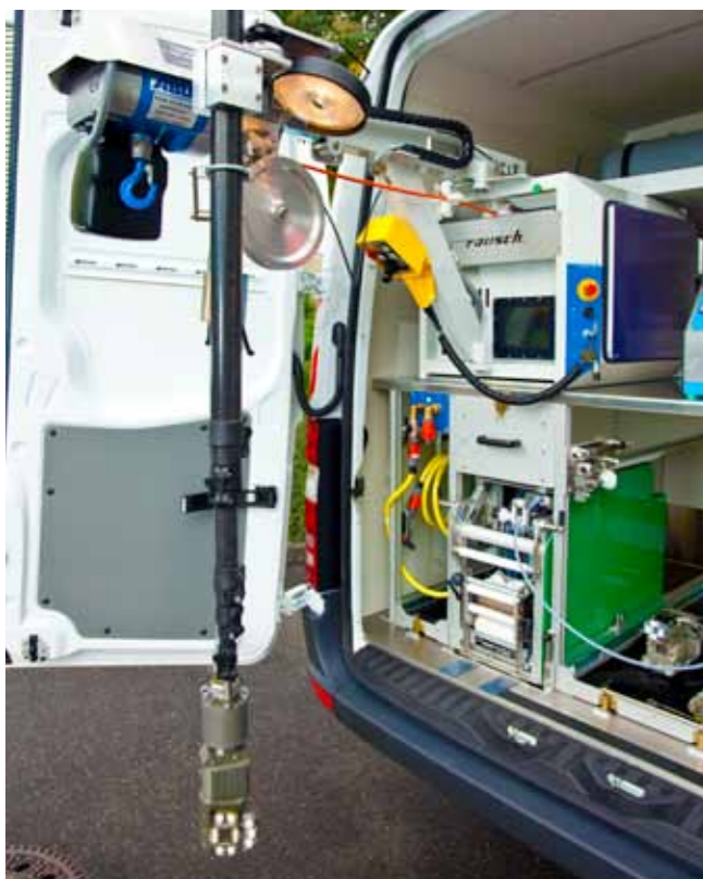
Manhole inspection with the main camera KS135 in accordance to EN13508-2. Camera guidance via a telescopic rod from the cable drum ELKA 600.
